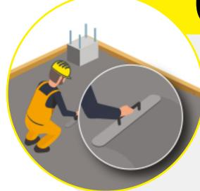
The last step is trowelling, in which the steel trowel is used.
