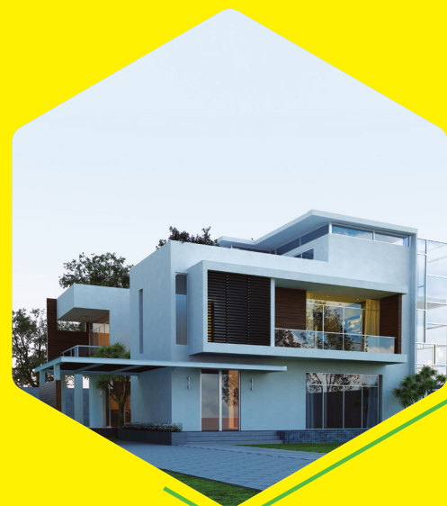
The multi-speciality concrete.
