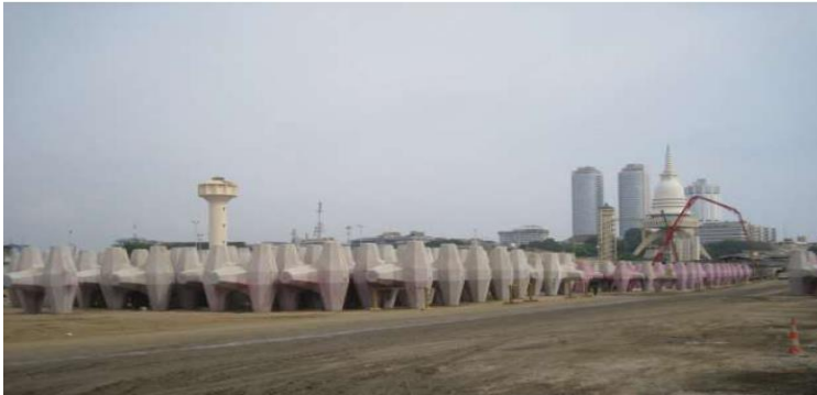
Expansion project at Port of Colombo
