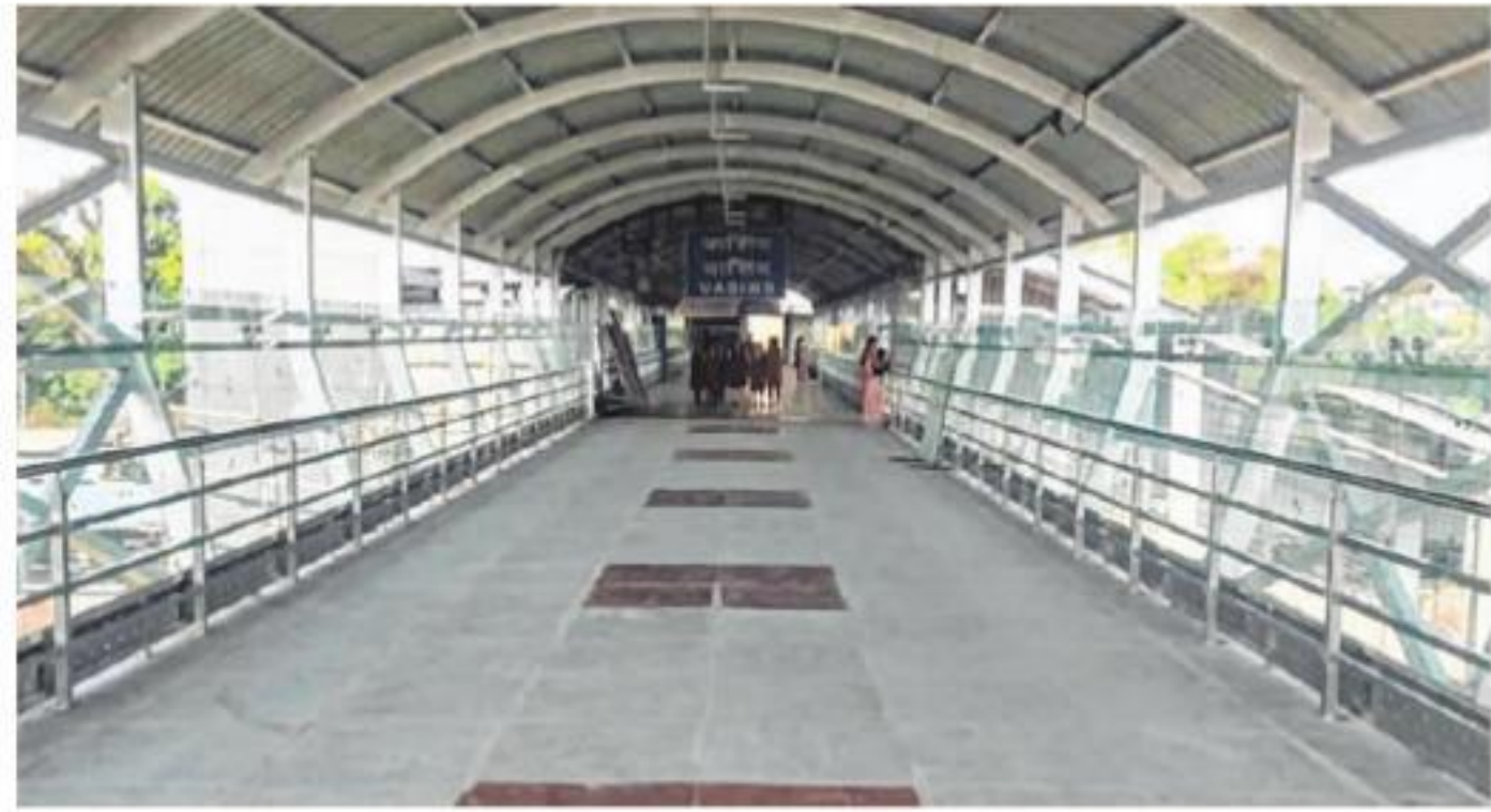
The work of a new foot over bridge (FOB), connecting the east side of the Vasind station with the UP line platform, has been finally completed. Spanning six metres in width and 30 metres in length, the connector has been built at ₹2.16 crore.
