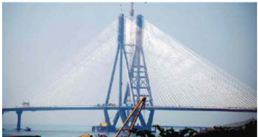
Grasim is the "Preferred Cement Supplier" for the Bandra-Worli Sea Link, an 8 lane, 5.6 km engineering marvel.
