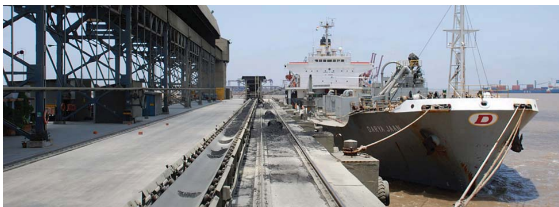
Jetty at Gujarat Cement Works
