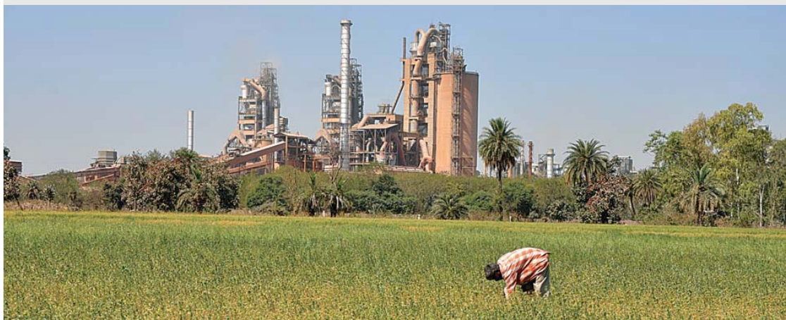
Limestone reject after screening is used as a pollutant absorber
