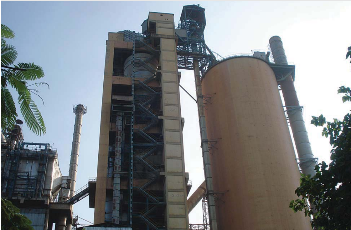
Many of our plants are designed to accept alternative fuels, such as Reddipalayam plant (above)
