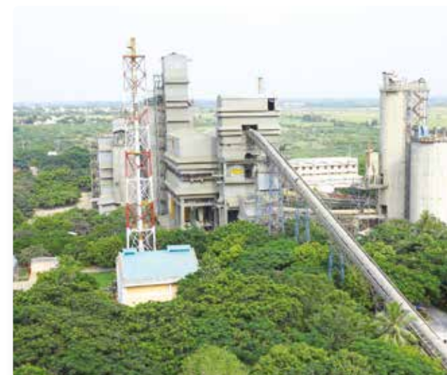
Arrakonam Cement Works
