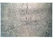
size aggregate shrinks more than concrete made with bigger size aggregate. The magnitude of drying shrinkage is also a function of the fineness of gel. The finer the gel the more is the shrinkage.
