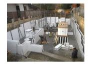
**6. Permanent Insulated Formwork Systems**: Insulating concrete forms (ICF) are typically used to construct permanent insulated formwork systems. Such formwork is usually assembled at the construction site. Once the concrete has been cured, this formwork stays in place. It is much stronger than other types of formworks and also enhances the speed of construction. Acoustic and thermal insulation offered by such formworks are higher compared to other types.
