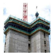
platform acts as a storage and distribution area while the middle platform, which is the main working platform, is at the top of the poured concrete level. The lower platform provides access for concrete finishing.
