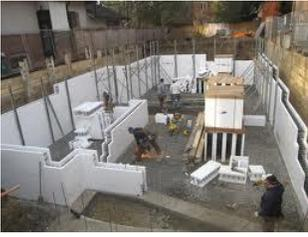
**6. Permanent Insulated Formwork Systems:** Insulating concrete forms (ICF) are typically used to construct permanent insulated formwork systems. Such formwork is usually assembled at the construction site. Once the concrete has been cured, this formwork stays in place. It is much stronger than other types of formworks and also enhances the speed of construction. Acoustic and thermal insulation offered by such formworks are higher compared to other types.
