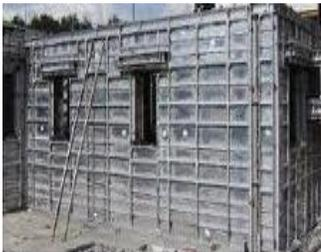
**2. Re-Usable Plastic/PVC/Aluminium Formwork Systems:** This type of formwork can be used repeatedly for constructing different types of structures/components. These systems are modular, interlocking and are simple to use as compared to other types. Houses built under mass housing schemes often utilize this type of formwork as they are robust and lightweight. They help to incredibly lower the cost of construction because of high number of repetitions possible.
